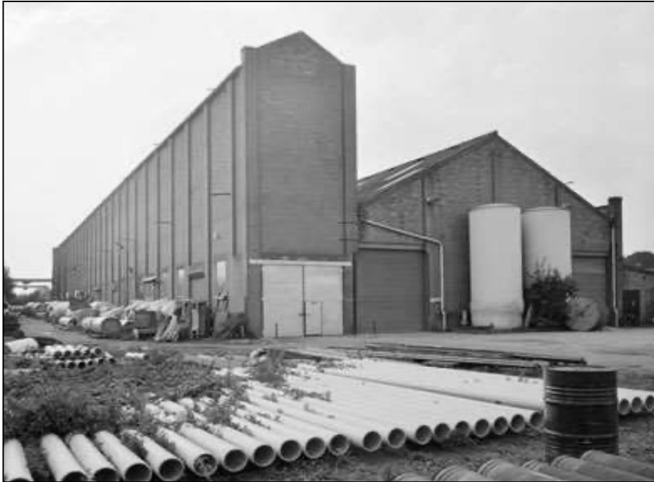
Royal Naval Cordite Factory, Dorset - Boiler and Generator House
