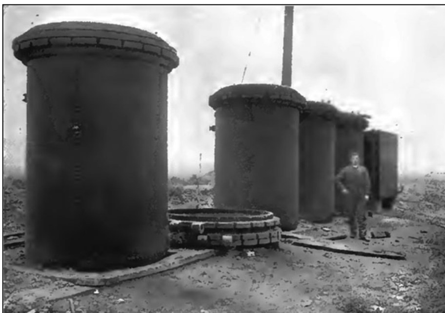
Fermentation VATS being erected at Rainham, Essex during the Autumn of 1912
