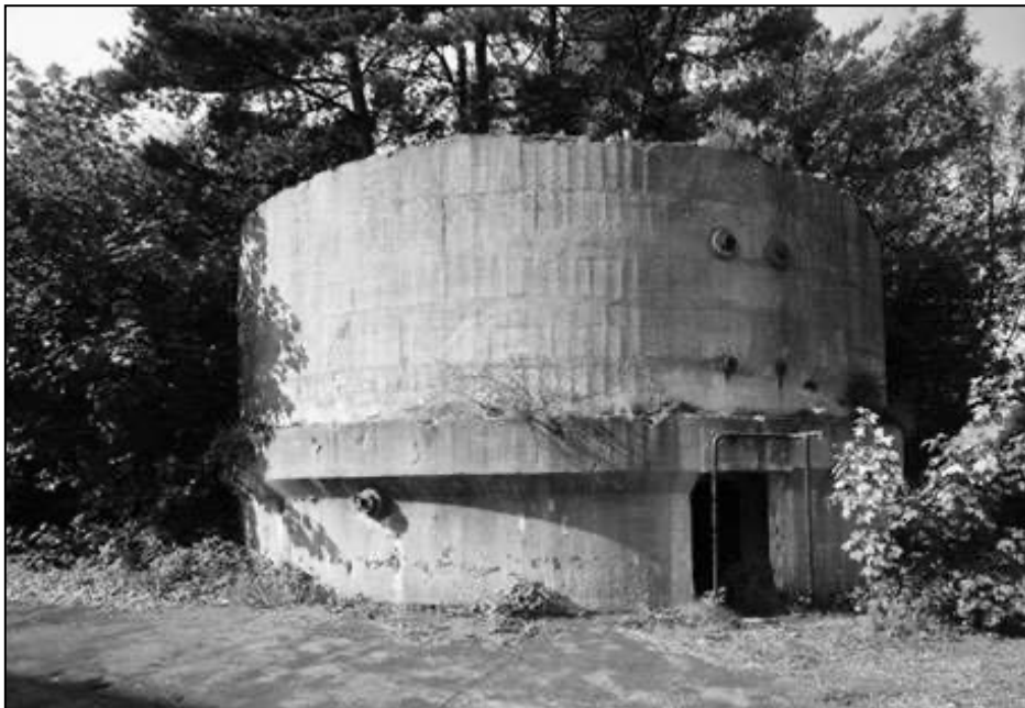
Royal Naval Cordite Factory, Dorset - Acetone Fermentation Tank
