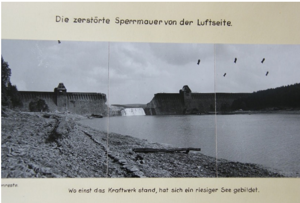
The destroyed one. The Dam barrier wall from the air (ground) side.
