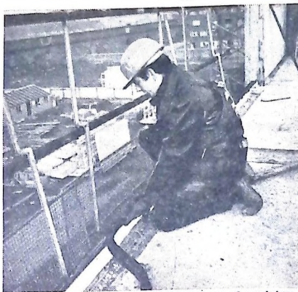
This picture shows the simple process of applying Compriband to form a watertight sealant between concrete slabs.
