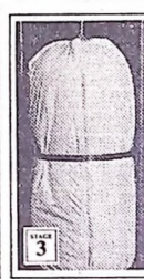
New hot water cylinder is fitted and lagged with special insulating jacket.
