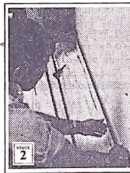
Pipe runs being laid (the small-bore pipe slips neatly through walls and fits snugly against skirting boards).
