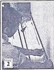
Pipe runs being laid (the small-bore pipe slips neatly through walls and fits snugly against skirting board).
