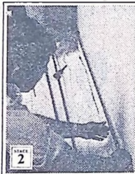
Pipe runs being laid (the small-bore pipe slips neatly through walls and fits snugly against skirting boards).
