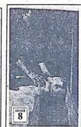
Roof insulation laid between rafters in attic space.
