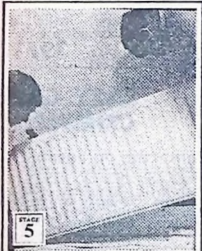
Radiators clamped in position and connected to pipes. There are 5 radiators in the package offer.
