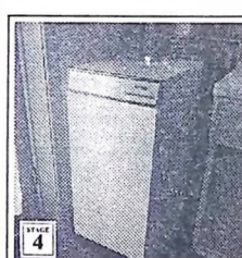
Boiler is secured in position.
