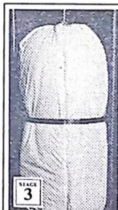
New hot water cylinder is fitted and lagged with special insulating jacket.
